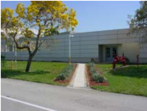
The walkway to building 99
