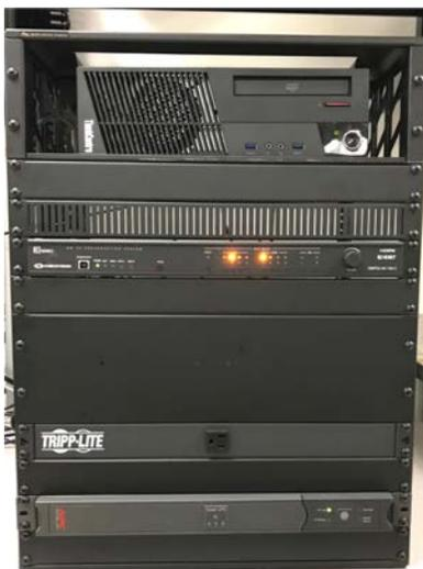
Typical rack installed in an approved credenza. The Credenza designed for multimedia components have necessary vents, power, space for equipment racks, and IR extenders (built in the furniture)
